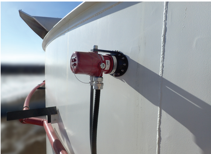
In this Zone 1 classified fixed-roof internal floating tank application, the optical flame detector is flange mounted. This installation technique allows for easier maintenance of the detector.
