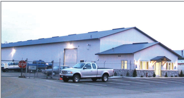
Det-Tronics Engineering Test Center Savage, MN
