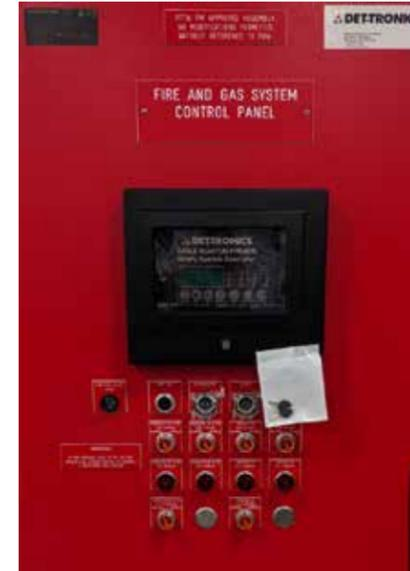
Listed fire and gas system components are performance-certified individually and as assembled systems.
