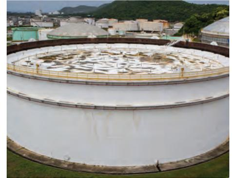
Around the world, there are over 4,800 oil terminals responsible for storing nearly a billion cubic meters of crude oil and other combustible or flammable petroleum products (source: [www.tankterminals.com](http://www.tankterminals.com)). Many of these terminals use floating roof tanks (FRTs). Though FRTs are considered safer than traditional fixed-roof and open-top storage tanks, they still afford the possibility of gas or vapor leaks that can ignite due to lightning or other causes.
